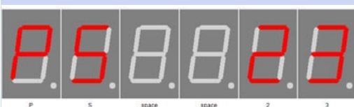
StandBy (Powersave) Start Hour
